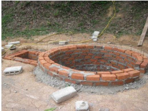
Fig. 12. Building the digester wall of a household unit using burnt-clay bricks
