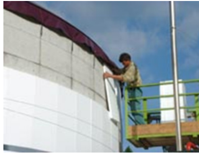
Fig. 17. Installing the insulation (BIOGAS NORD GmbH)
