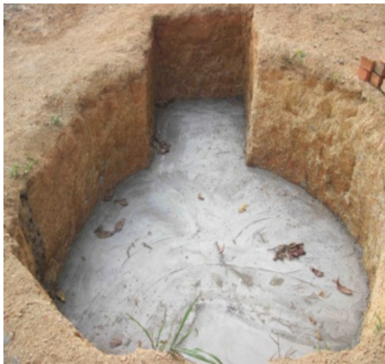
Fig. 10. Concrete bottom of a household unit
