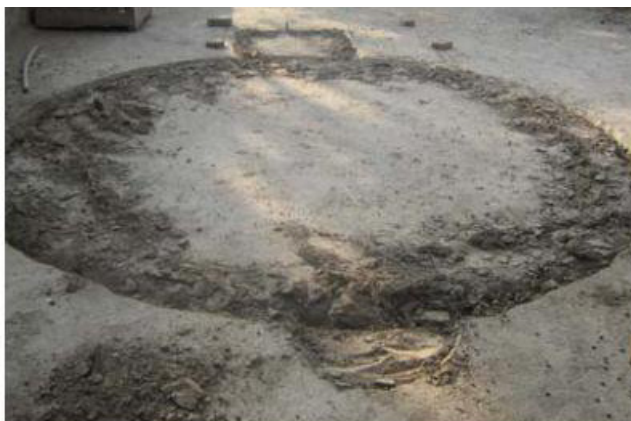
Fig. 5. Marking of dimensions for a biodigester
