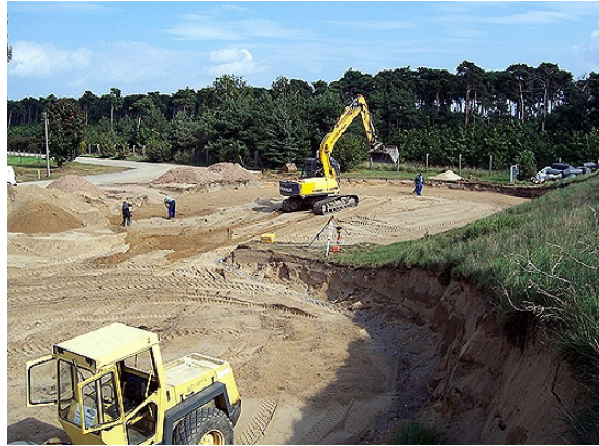
Fig. 7. Excavation works for a commercial biogas plant
