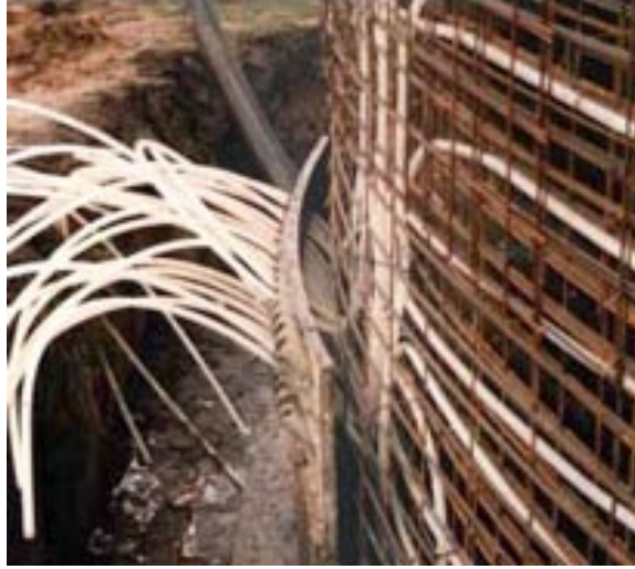
Fig. 13. Integrating the heating tubes (BIOGAS NORD GmbH)
